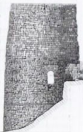
Anacopia tower. East facade. Restoration
